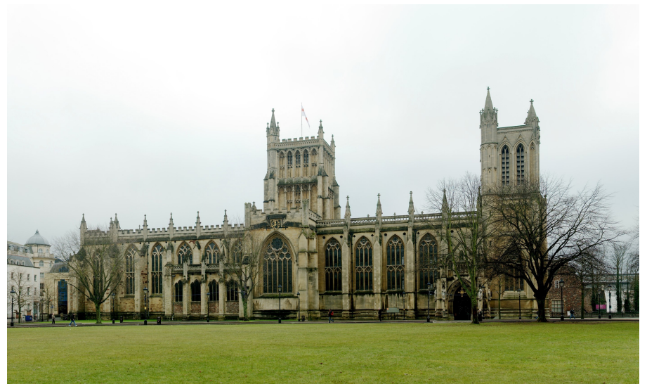
The Cathedral Church of the Holy & Undivided Trinity, once St Augustine's Abbey, seen across College Green, so named after Robert Fitzharding's College of canons.
