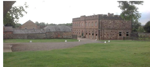
The Berkeley Hunt stables and kennels
